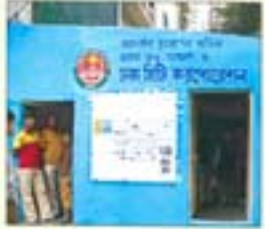
Ward Office Renovation (February 2008)
